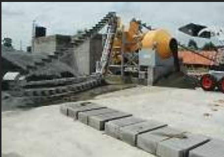
BATCHING PLANT TRAINING
